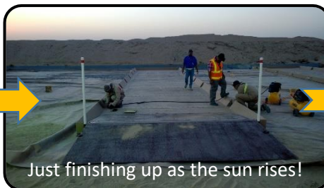
Construction starts after dark due to hot desert days ...
