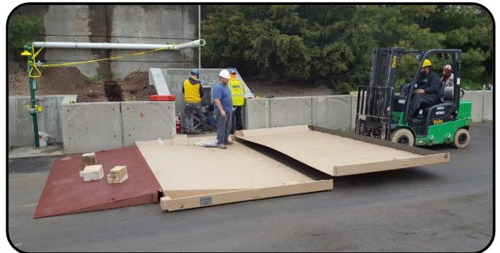
OVERLAPPING JOINT IS NEARLY FLUSH FOR SMOOTH RIDE ACROSS DECK. PROVEN DESIGN, NO LEAKS!
